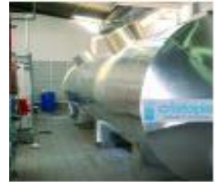
STL tank with Nodules (Encapsulated Phase change Material) Source: Cristopia.
